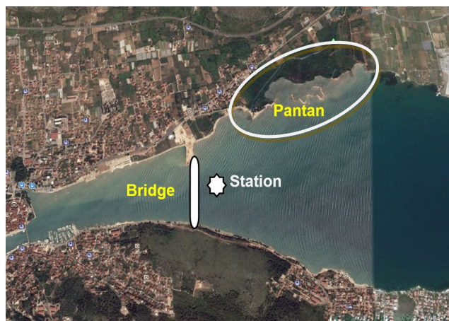
Figure 1: Location of bridge, Pantan area and measuring
